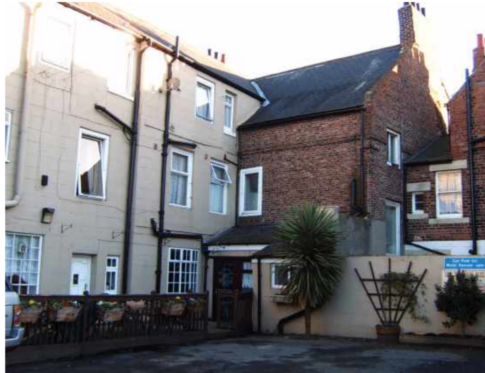
JUNCTION BETWEEN EARLY AND LATE GEORGIAN BUILDINGS
