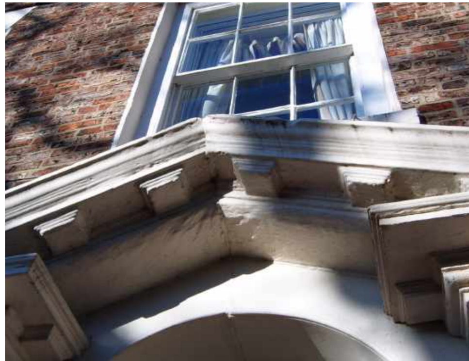
DETAILED VIEW OF THE MAIN ENTRANCE PORTICO
